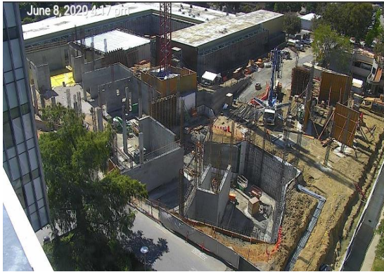
Figure 4. An image of the construction site investigated for this study.
