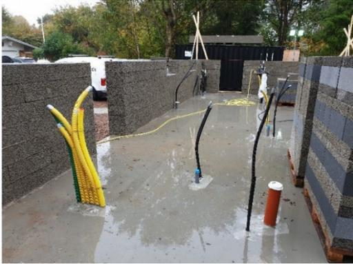
Figure 4. Typical small house slab cramped with construction material and cabling
