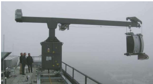
Figure 5. A robot with a rooftop gantry [16]
