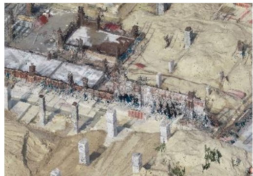
Figure 11. 3D point cloud model of the under-construction foundation work.
