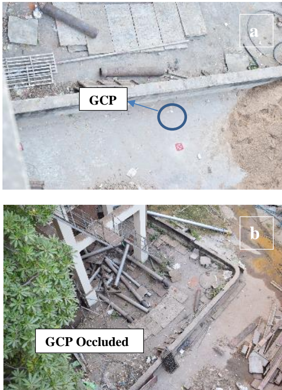
Figure 4. (a) Marked GCP at construction site and (b) GCP occluded due to site activities.
