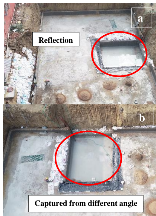
Figure 9. (a) reflection due to water (b) reflection avoided by trajectory modification
