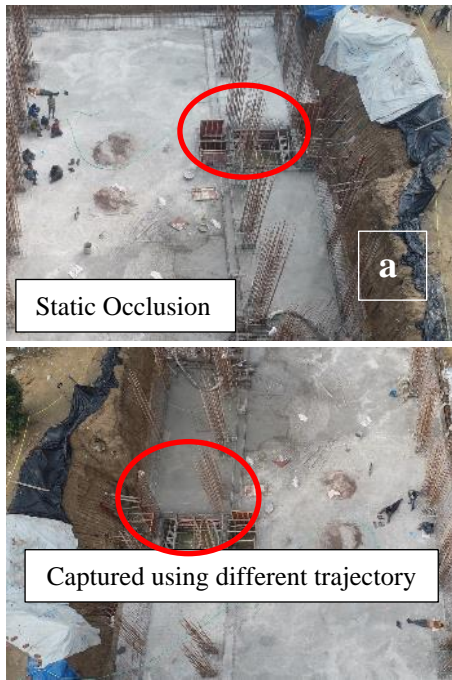
Figure 5. (a) Occlusion due to structural component, (b) occlusion avoided using different UAV trajectory.
