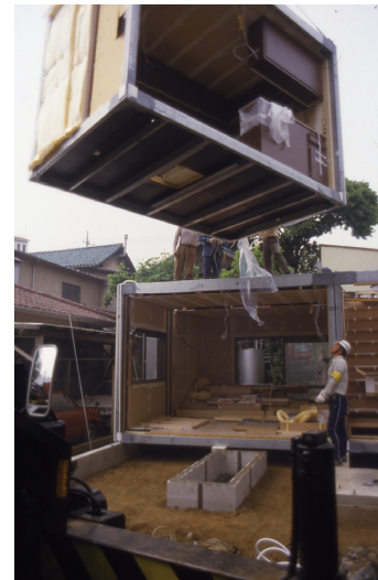
Figure 4: Transport of completed Units from the factory to the site
