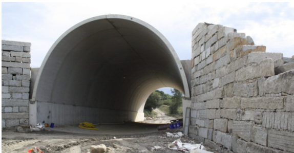
Fig.1. Underpass arch-shape structure, under survey in the highway Ourense-Celanova before filling and structural settlement.
