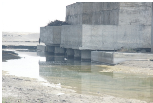
Fig.2 Exposed Pile Foundations
