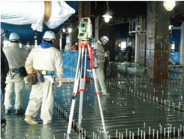
Fig.15 Field Test on the Construction Site (No.1)
