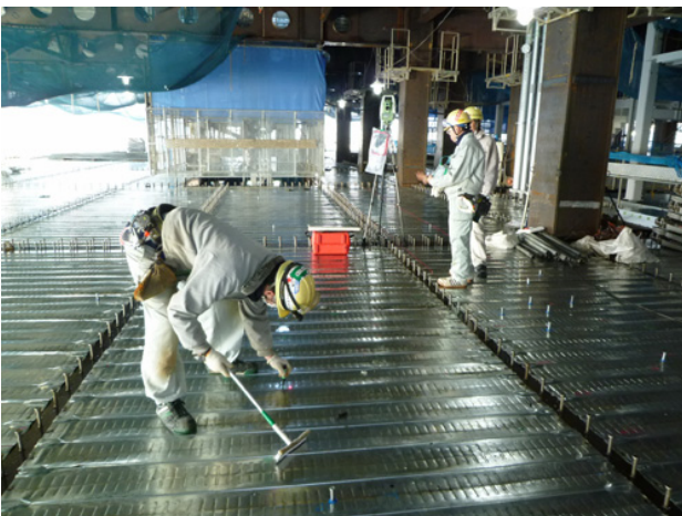
Fig.16 Field Test on the Construction Site (No.2)
