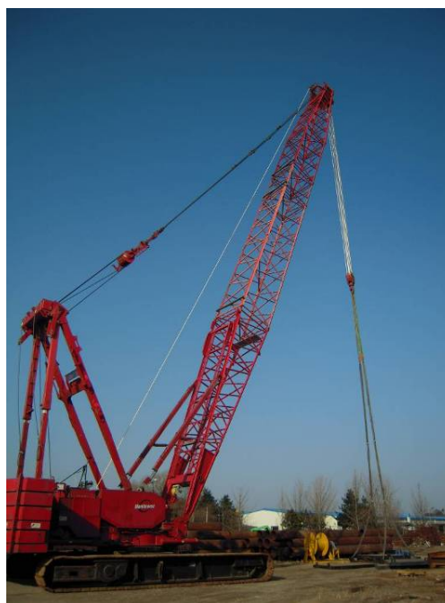
Fig. 6 Crane setup for the winding up test
