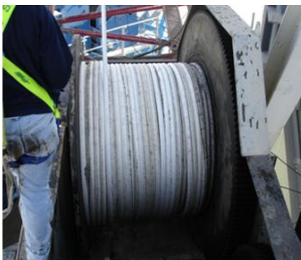
Fig. 3 Improper winding of the fiber rope
