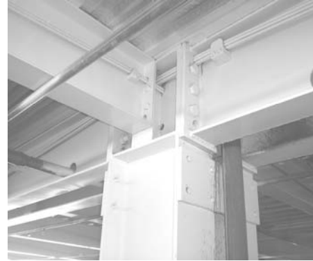
Figure 5: Post-tensioning cables at column junction
