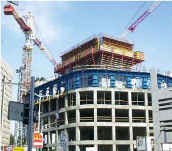
Figure 2. Field study building.
