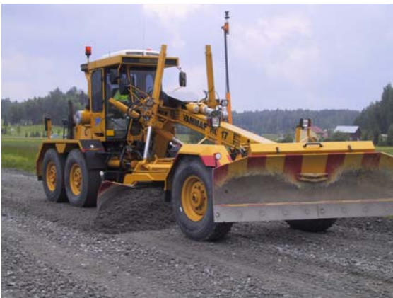
Figure 5. Automated control system of road graders on a motor way construction site, Salo, Finland, 2002.
