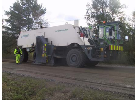
Figure 7. The real milling machine in the field tests (Figure: Andament Ltd).
