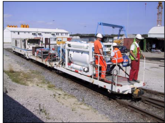
Figure 6: Transport Capsule to the TBM
