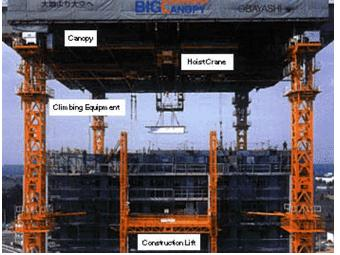
Fig. 2. Big Canopy automated construction system
