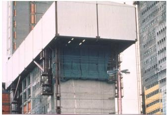
Fig. 1. Delftse Poort Mechanised Construction System
