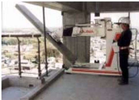
Fig.1 Wall Panel Handling Robot commercialized by Kajima
