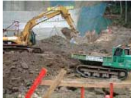
Fig.6 Excavation and loading by remote controlled excavators and crawler carriers.
