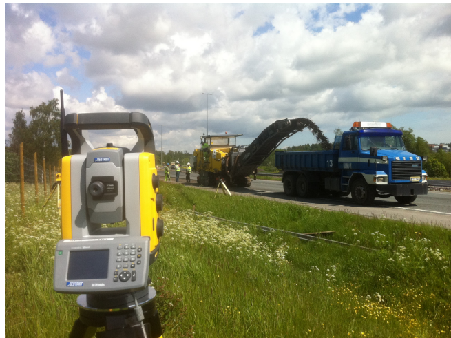
Figure 7. BIM based automated control of milling machine (robotic total station was used for 3D positioning, Trimble GSC900 system for the machine control).
