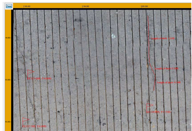
Fig. 8. Zoom-in at some crack locations of a bridge in New Jersey.
