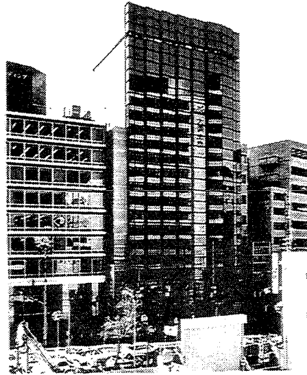
Building name: Yanagibashi Mitui Building Location: Nakamura-ku Nagoya, Japan Building area: 682.880 m 2 Total floor space: 7,940.822 m 2 Structure: RC, SRC, S structure Scale: B2F, 12F, P1F Maximum height: 44.95 m Construction period: Nov.1989- Feb.1991
