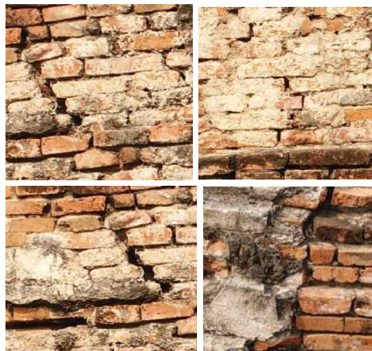
Figure 3 :Sample images of cracks in masonry structures
