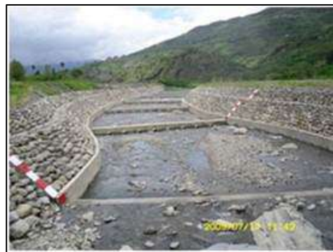
Figure 3. Groundsill works
