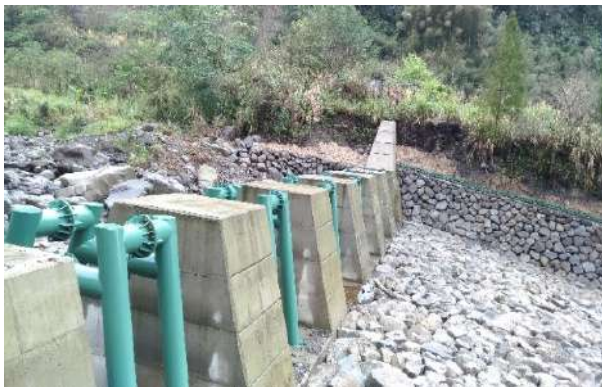
Figure 7. Steel-pipe-type slit dam of the case project
