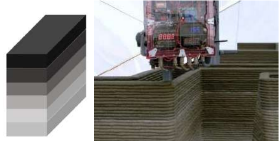
Fig. 6 left: Approach of CONPrint3D ® right: Extrusion of smaller concrete strands with round corners and subsequent concrete filling [8]
