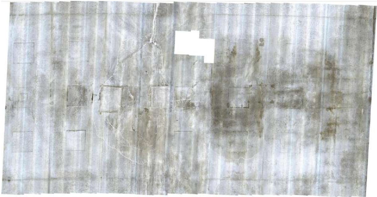
Figure 7. Panoramic texture image of a tunnel lining concrete made by NATM method
