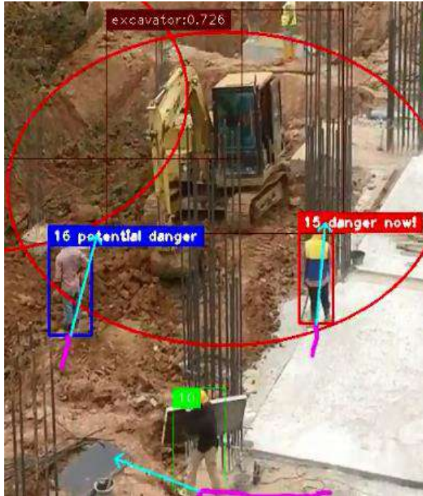
Figure 5. Examples of identified danger zones and different safety statuses of workers
