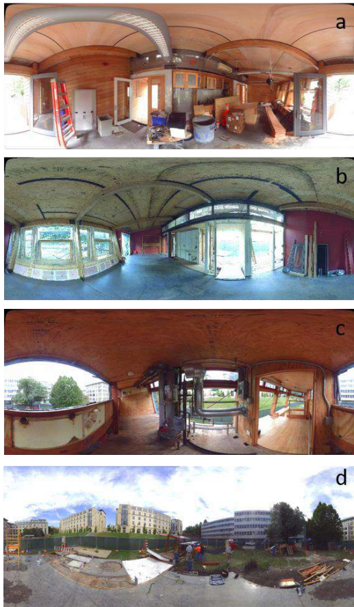
Figure 3. Point clouds captured at different times during the project: (a) before deconstruction, (b) after removing furniture and exterior walls, (c) after removing door and window frames, (d) after lifting the roof
