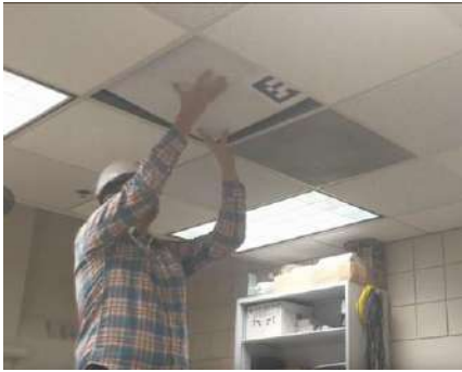
Figure 1. The construction process involves repetitive tasks with different objects, such as ceiling tile installation, the tiles are maneuvered and placed repetitively at different locations.
