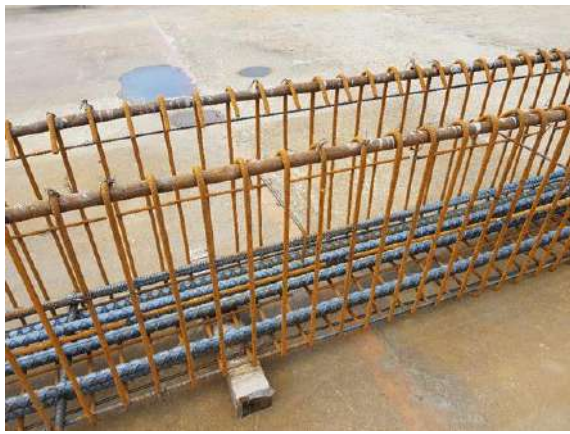
Figure 6. Stirrups of the precast beam.
