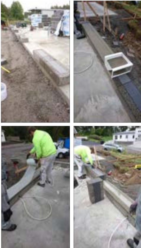
Figure 2. Steps in the masonry process with Finja Exakt block system; first layer (top left), application of mortar (top right), application of reinforcement (bottom left) and customization for cabling (bottom right).
