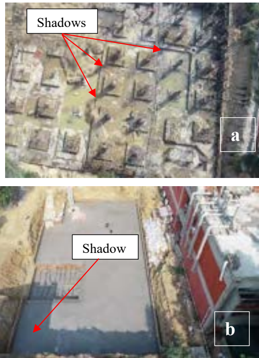
Figure 10. (a) Multiple shadows due to structural elements (b) Shadows due to adjacent structures
