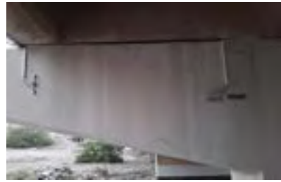
Figure 6. Mechanical remote sensors for bridge data collection
