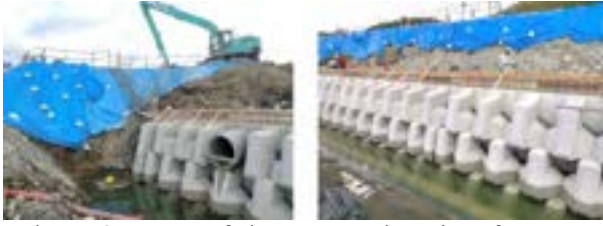
Figure 9. Scene of the construction site of wave-dissipating block installations at Toyoura coast
