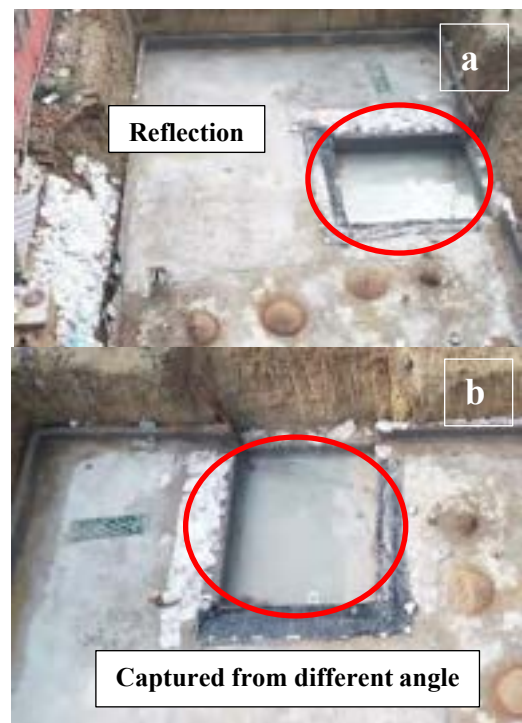
Figure 9. (a) reflection due to water (b) reflection avoided by trajectory modification
