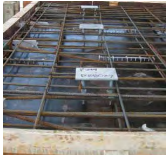
Figure 3. Formwork, rebar, and embeds positioned prior to concrete pour.
