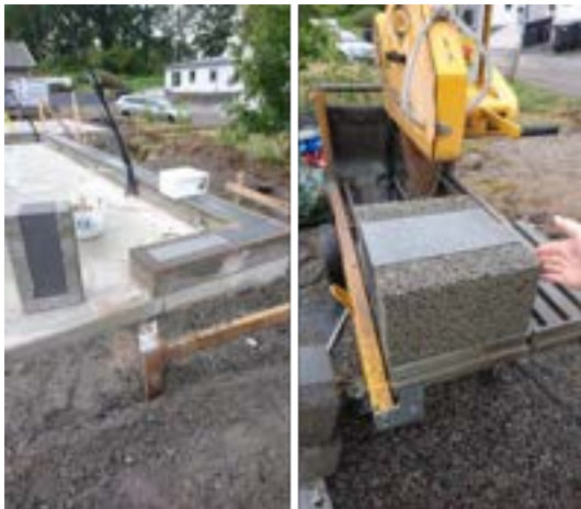
Figure 3. Finja Exakt Block with corner block (left) and on-site customization of sawing block (right).
