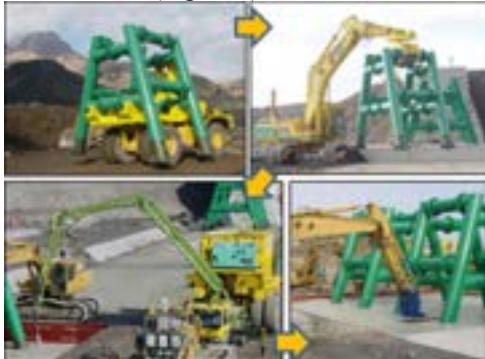
Figure 5. Building of a steel slit dam
