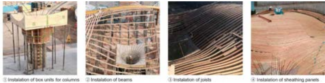
Figure 2. Work procedure of formwork for Kawaguchi project's free-form roof
