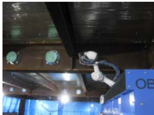
Figure 4. Steel Girders and Beams Before Spraying
