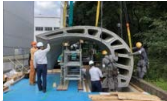
Photo 10. Erection and installation of the pieces
