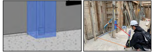
Figure 7. BIM model reference (left) and actual environment (right).
