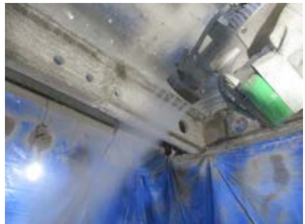
Figure 3. Dust Scattering Prevention Nozzle
