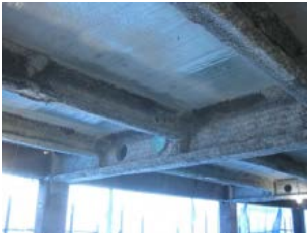
Figure 9. Girders and Beams After Sprayed
