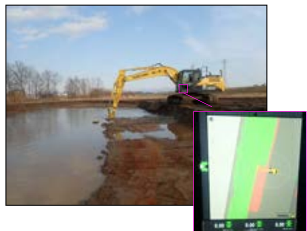
Figure 5. ICT construction (3D-machine control) (Appearance Guidance and the monitor which shows the excavation status in operation room)
