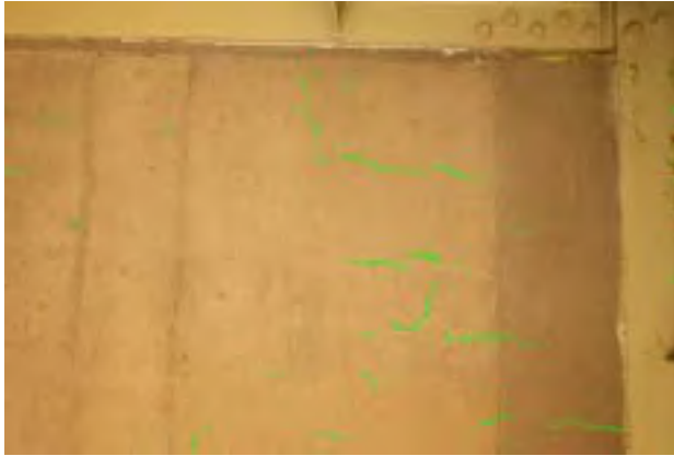
Figure 4. Bridge deck crack extraction image
