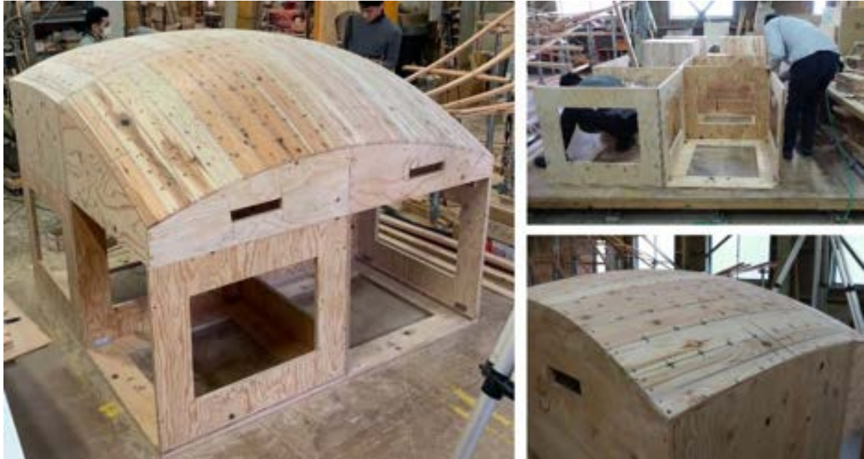
Figure 5. New Method's formwork unit
