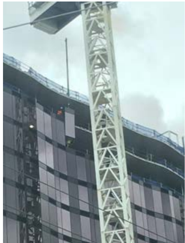
Figure 3. Direct conventional UCW installation method: Transitioning from the vertical transport task to the alignment task (photo by B. Johns, 2019)
