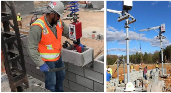
Figure 1. Human-robot collaboration on the construction jobsite using a masonry robot [22].
