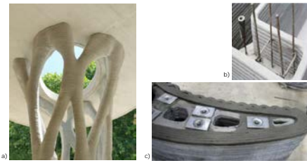
Figure 2. Post-reinforcement: a) Pile with printed formworks [10] b) traditional reinforcement [2] c) reservations for prestressing cables [21]
