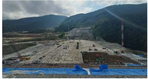
Figure 3. Overlook of autonomous construction of Naruse Dam in Japan.[20]
