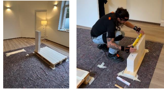
Figure 4. First process variant, human-based, manual (left: setup, right: MoCap recordings)
